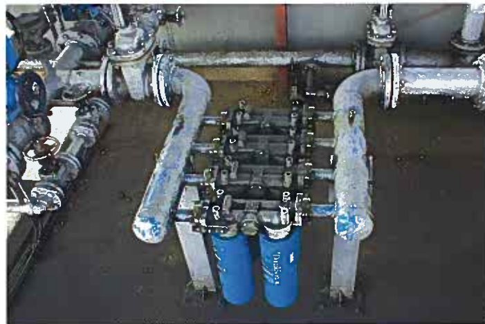
Donaldson recommends using spin filters for bulk biofuel filtration
